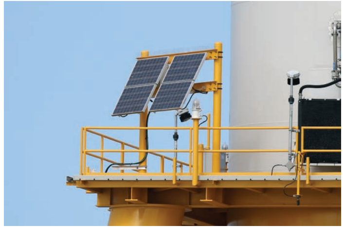
Offshore Wind Farm
