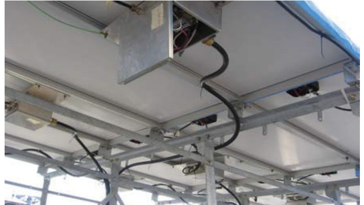
Heavy Duty Interconnection between Solar Modules
